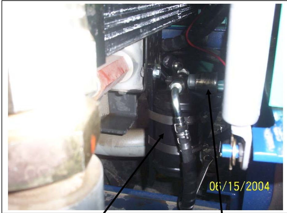
Receiver drier assembly
