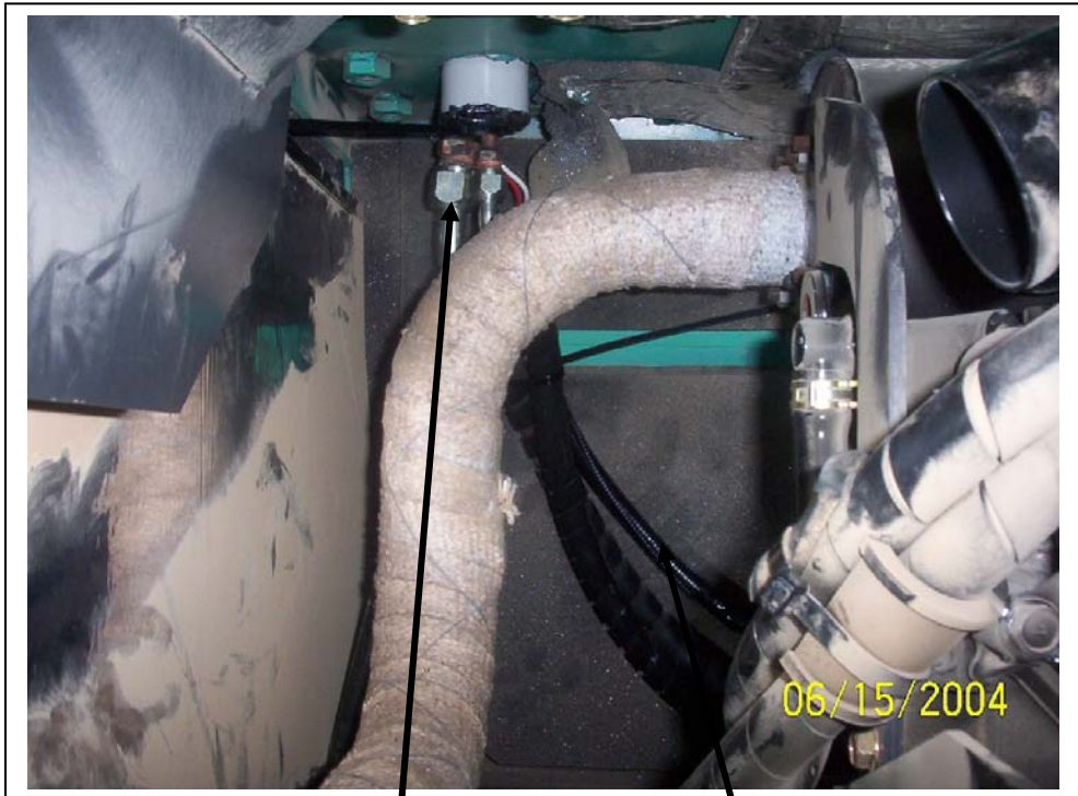
Connections under cab
